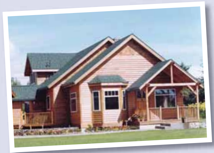
The Sughrue home in Vancouver, Washington, integrates SIPs and recycled timbers for energy and resource efficiency. Built in 1999, heating bills have averaged only US$350 per year.
