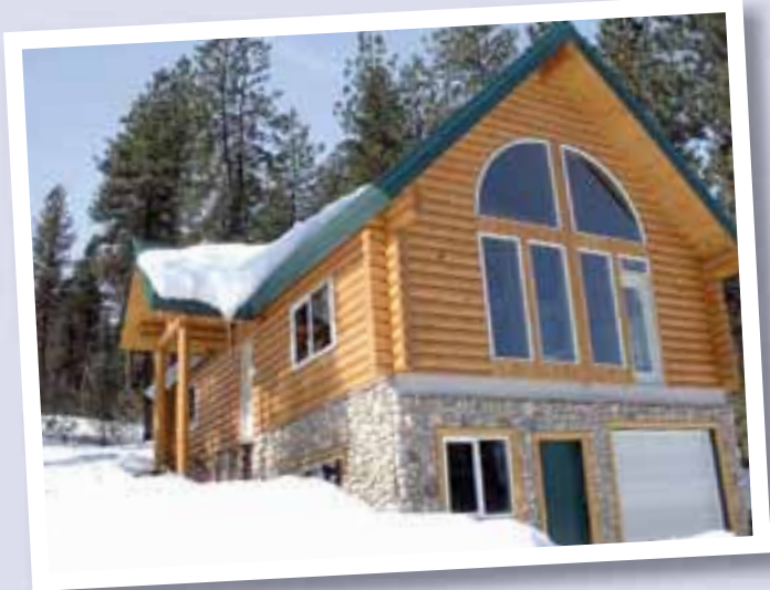
With logs having an insulation value of only R-1 per inch of wood, adding SIPs to the roofing system of this home makes the whole building more efficient.
