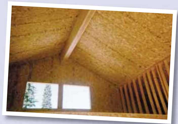
Versatile SIP gable walls and roofs can accept a variety of interior finishes.
